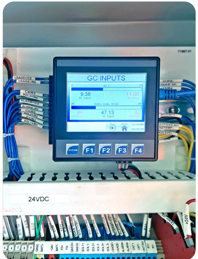
Figure D9. Welker PLC at 10% stage.
