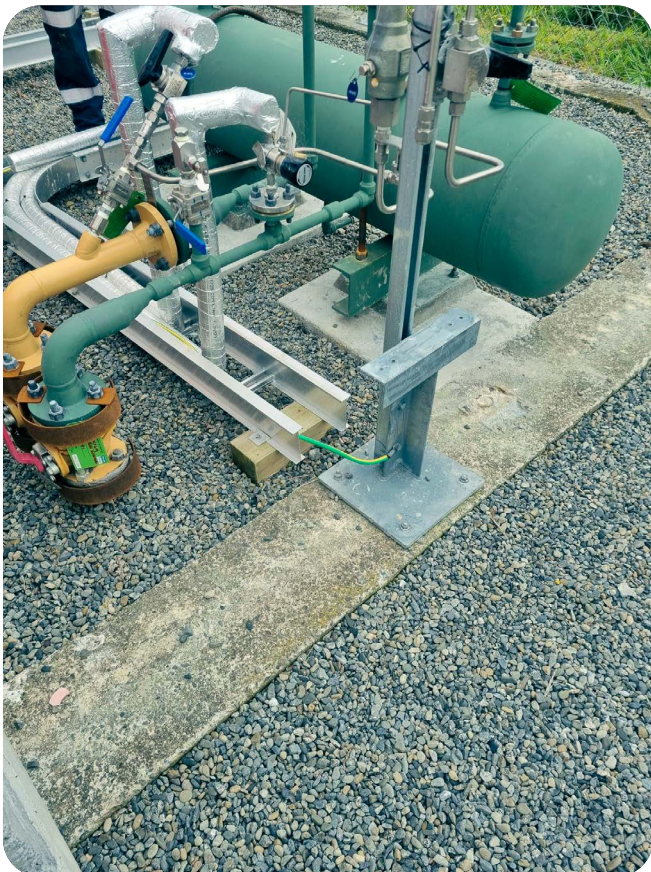
Figure D7. H 2 mixing loop with tank.
