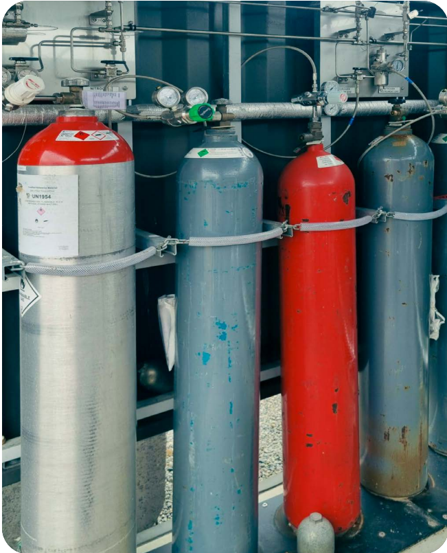
Figure D5. Welker H 2 injection & GC calibration cylinders at the DP.
