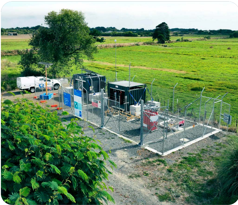
Figure D1. Te Horo DP set up.
