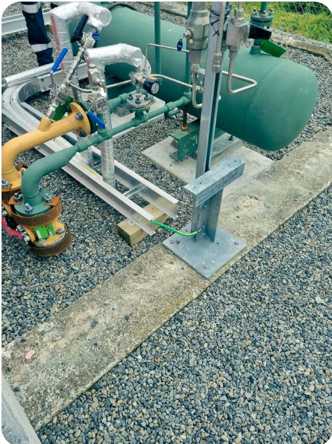
Figure D7. H 2 mixing loop with tank.
