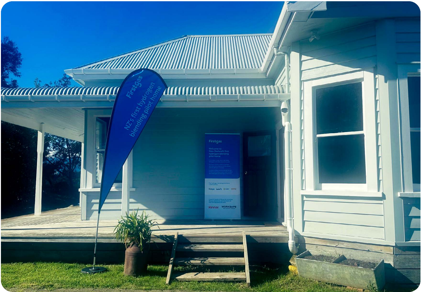
Figure D10. Firstgas hydrogen display home.
