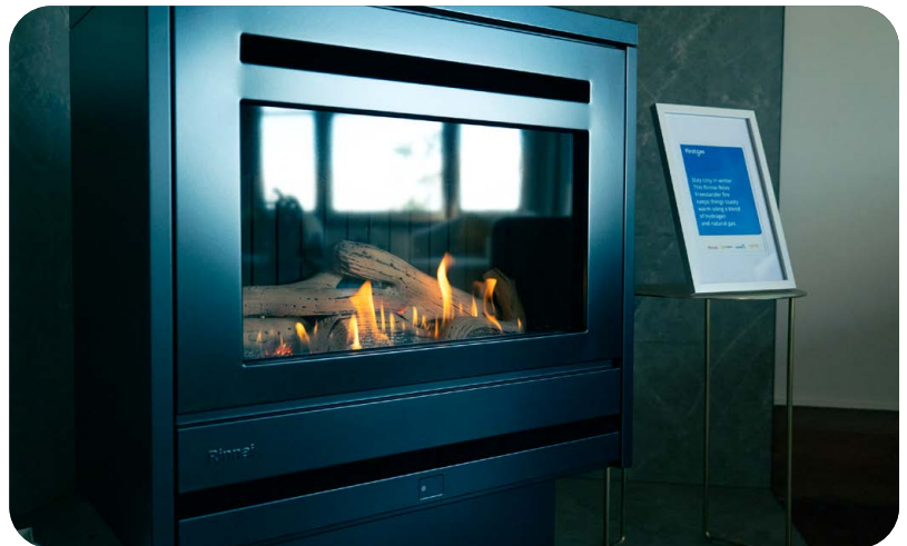
Figure 7. The Rinnai gas heater running on a hydrogen blend in the display home
