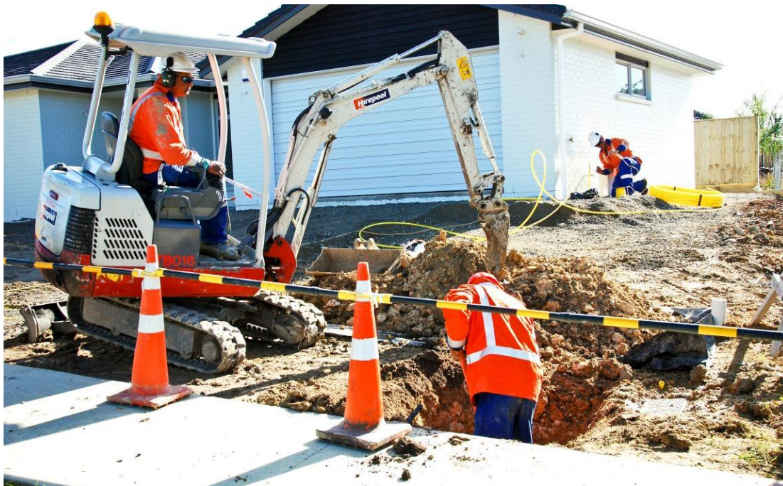
Figure 19: Installation of a New Customer Connection
