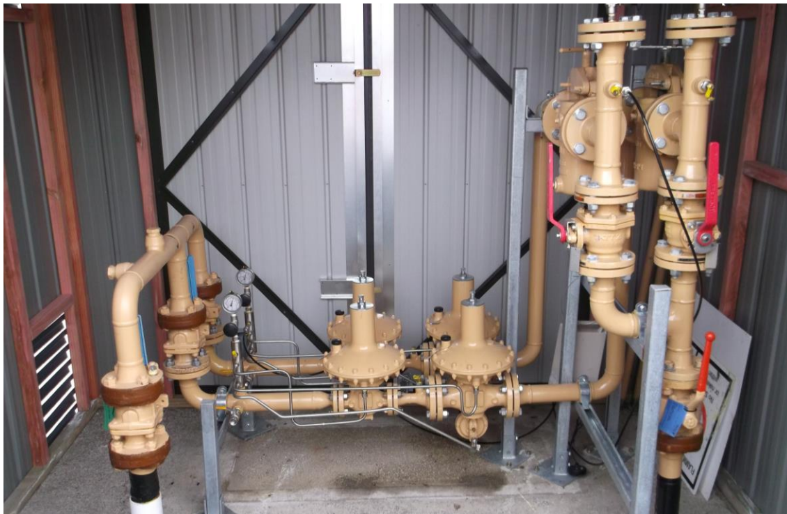
Figure 12: A standard DRS installation
