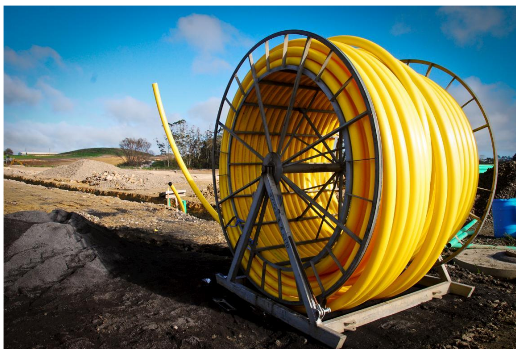
Figure 11: Typical PE mains pipe installation
