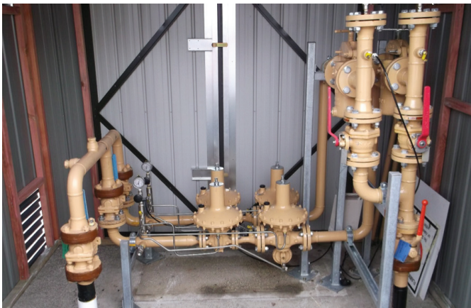
Figure 19: A standard DRS installation
