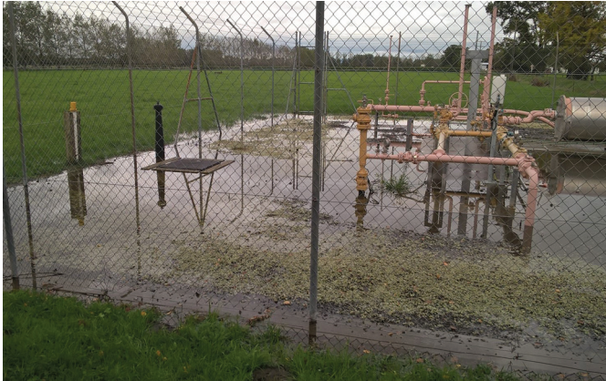
Figure 12: DRS 80247 Waitoa submerged under water contrasted with DRS unit lifted above ground
