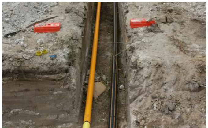
Figure 11: Relocated distribution steel and new PE pipes
