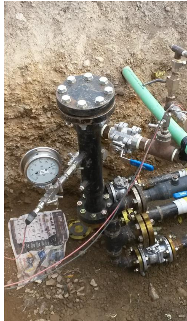
◀ The picture shows a planned hydrotest of the distribution system to confirm the allowed operating pressure.
