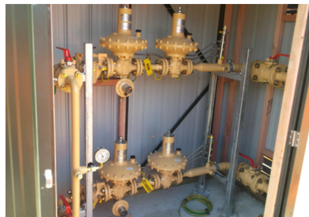
◀ The picture shows a typical district regulator station in an above ground enclosure.
