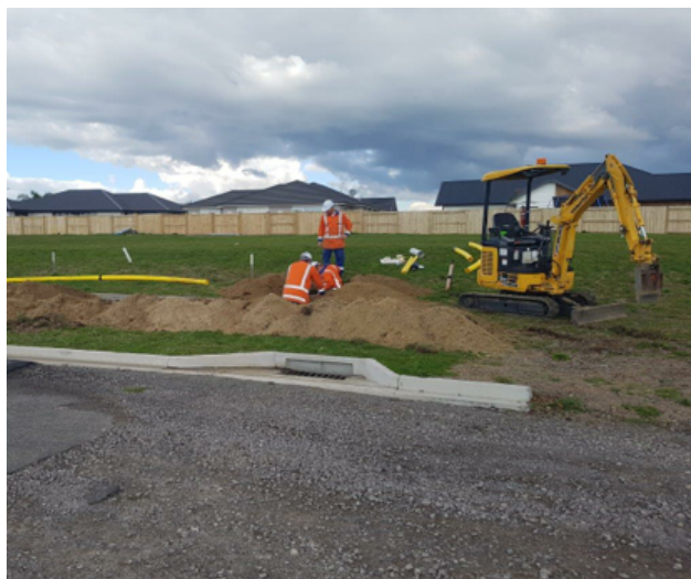
◀ The picture shows gas distribution mains construction at new Papamoa development sites.
