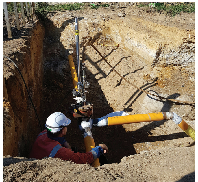
▲ This picture shows the new IP20 steel tie into existing IP20 gas pipeline in Cambridge
