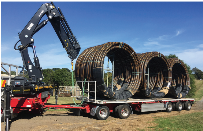
▼ Rolled PE mains delivered on site
