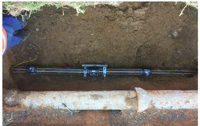
▼ New PE pipe in the ground
