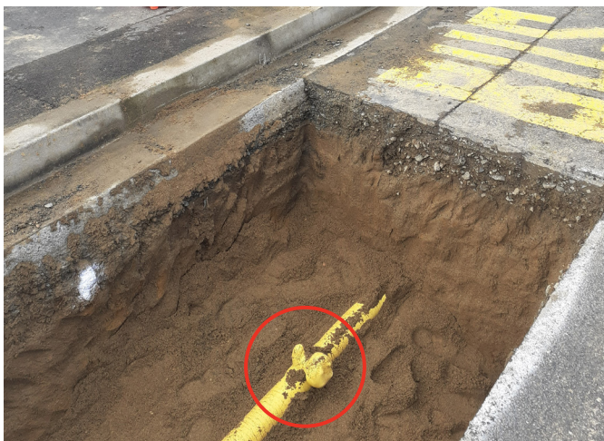
Figure 9: Pre-1975 pipeline remediation, Hamilton (Pre-1975 off take section was removed and decommissioned)
