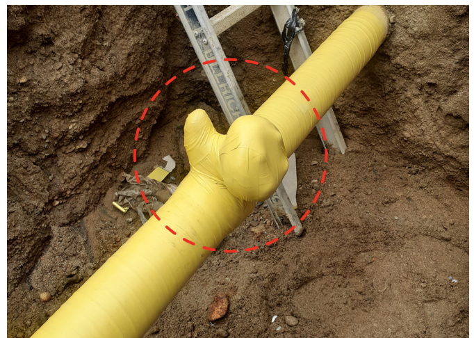
Figure 9: Pre-1975 pipeline remediation, Hamilton (Pre-1975 off take section was removed and decommissioned)
