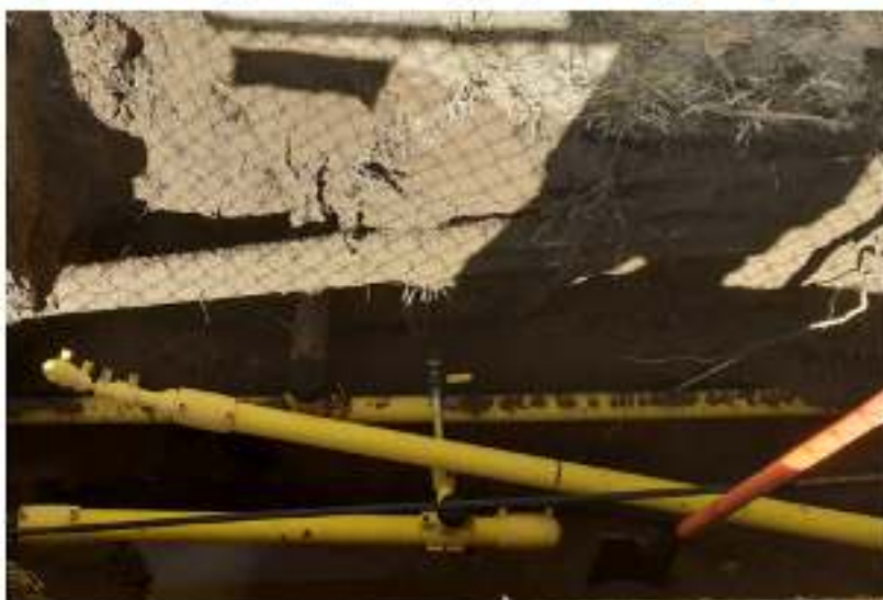
Figure 1: Pre-1985 pipeline replacement project, with new PE pipe being installed
