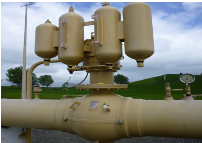
Figure 23: Typical manually operated MLV
