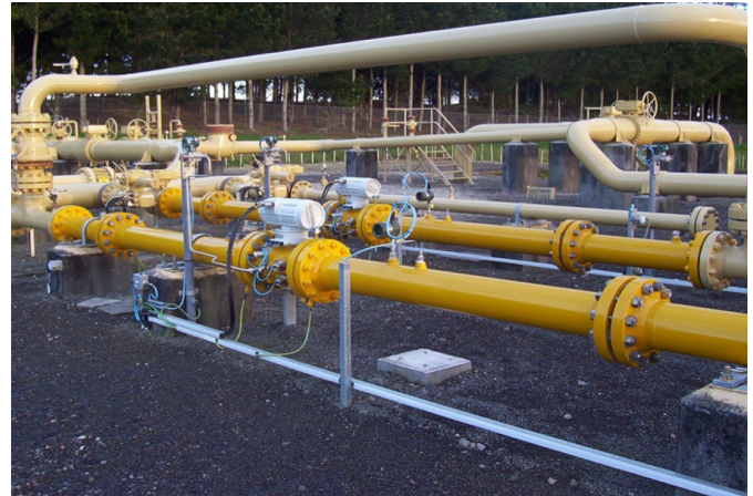
Figure 32: Typical ultrasonic metering system
