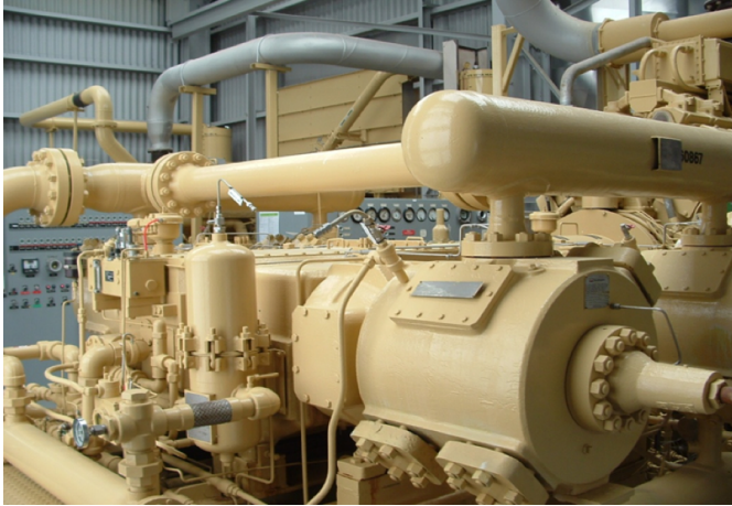
Figure 25: Typical reciprocating gas compressor
