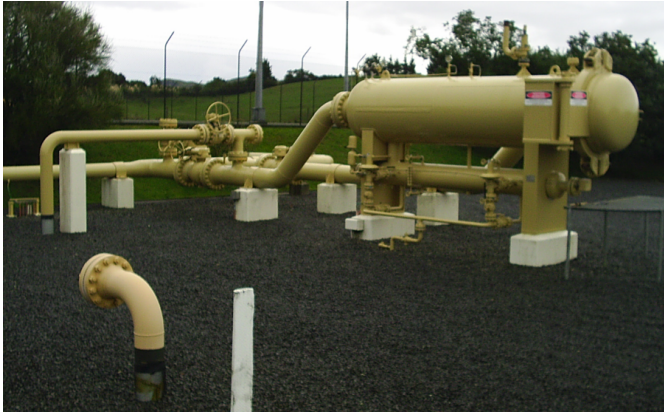
Figure 28: Typical filter separator
