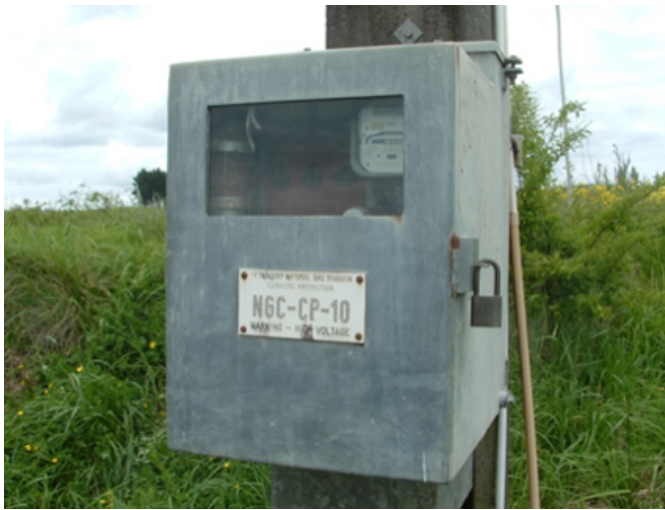
Figure 21: Typical pole mounted rectifier unit
