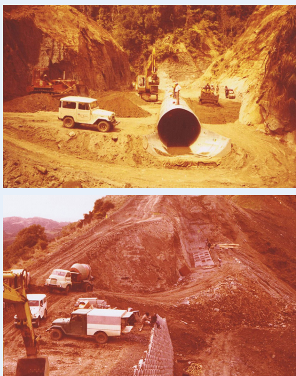
Figure 4: Pipeline construction circa 1977
