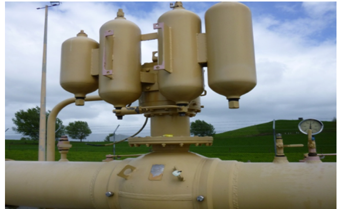
Figure 8: Typical manually operated MLV
