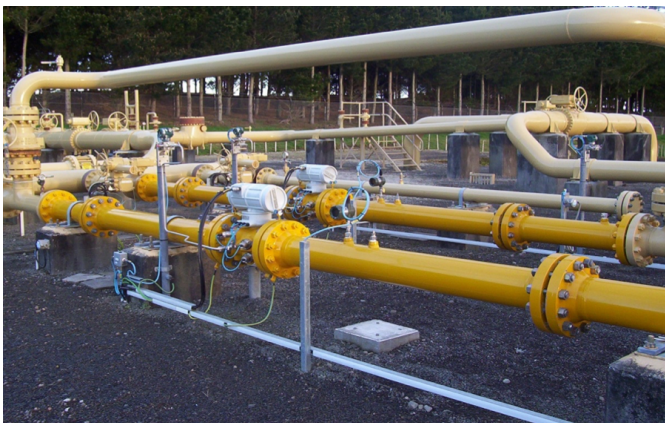
Figure 18: Typical ultrasonic metering system
