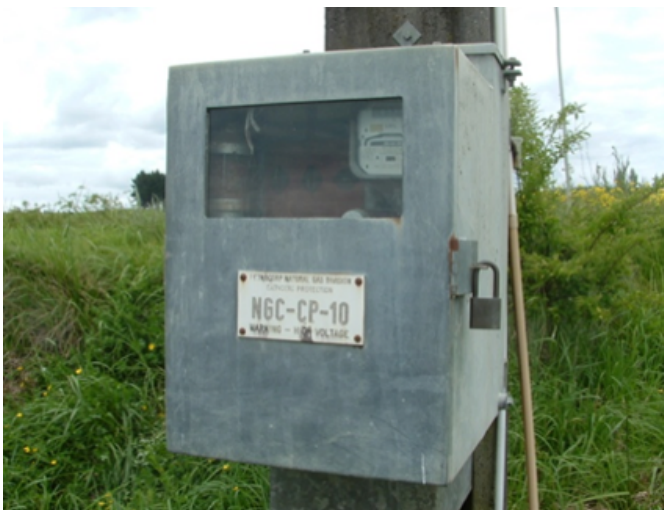
Figure 6: Typical pole mounted rectifier unit
