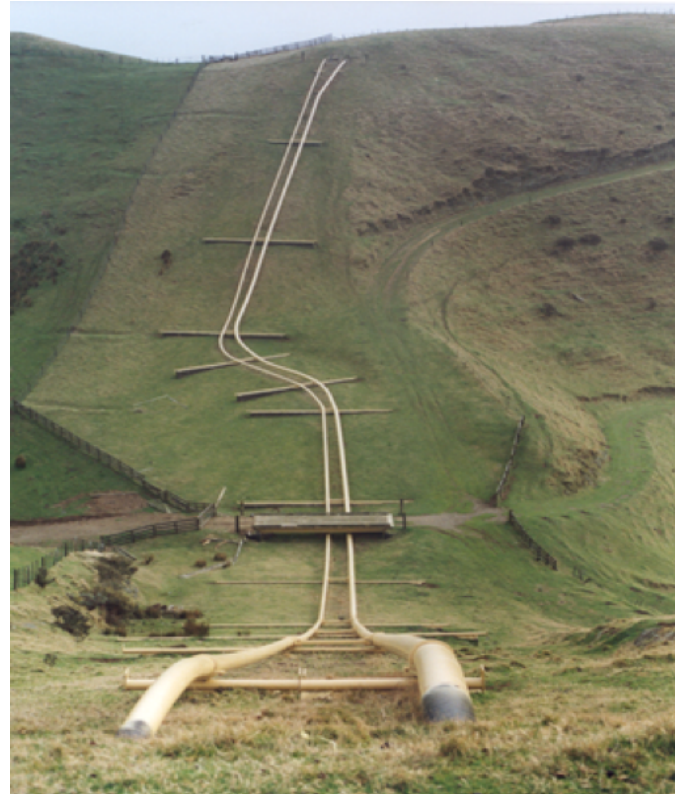
Figure 4: Pipelines at Gibbs Fault near Wellington
