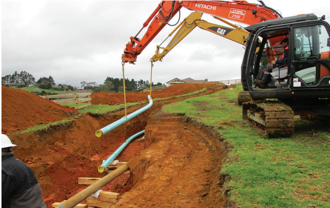
Figure 12: 200 line realignment at Runciman Road
