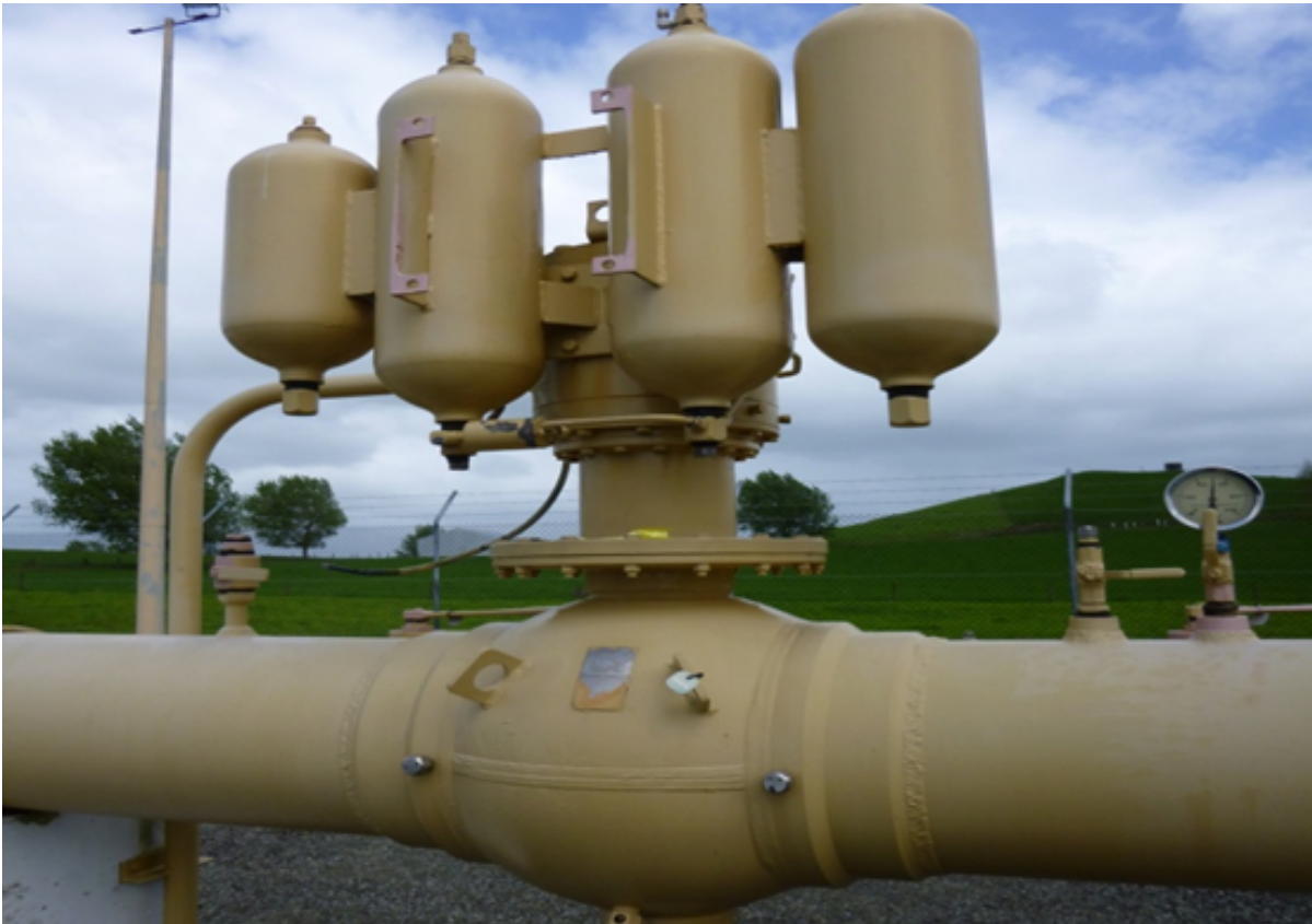
Figure 23: Typical Manually Operated MLV
