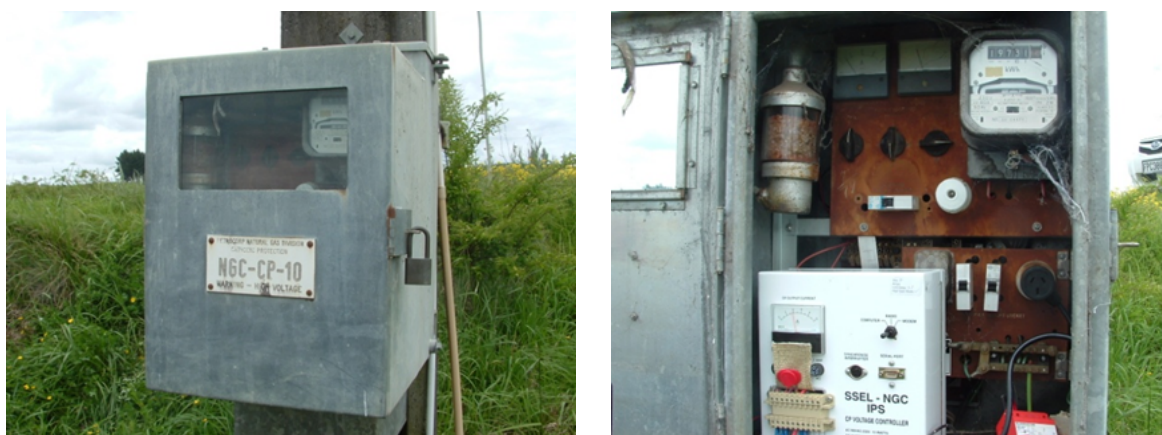
Figure 21: Typical pole mounted rectifier unit
