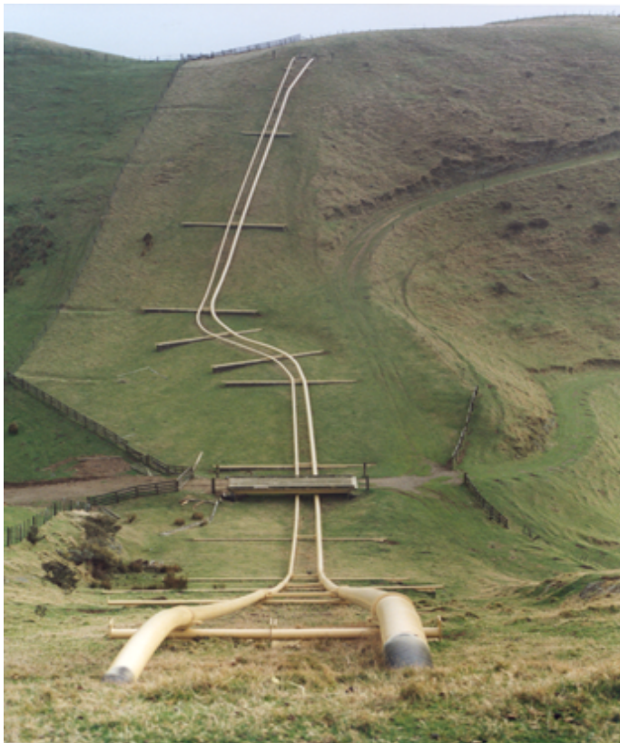
Figure 19: Pipelines at Gibbs Fault near Wellington
