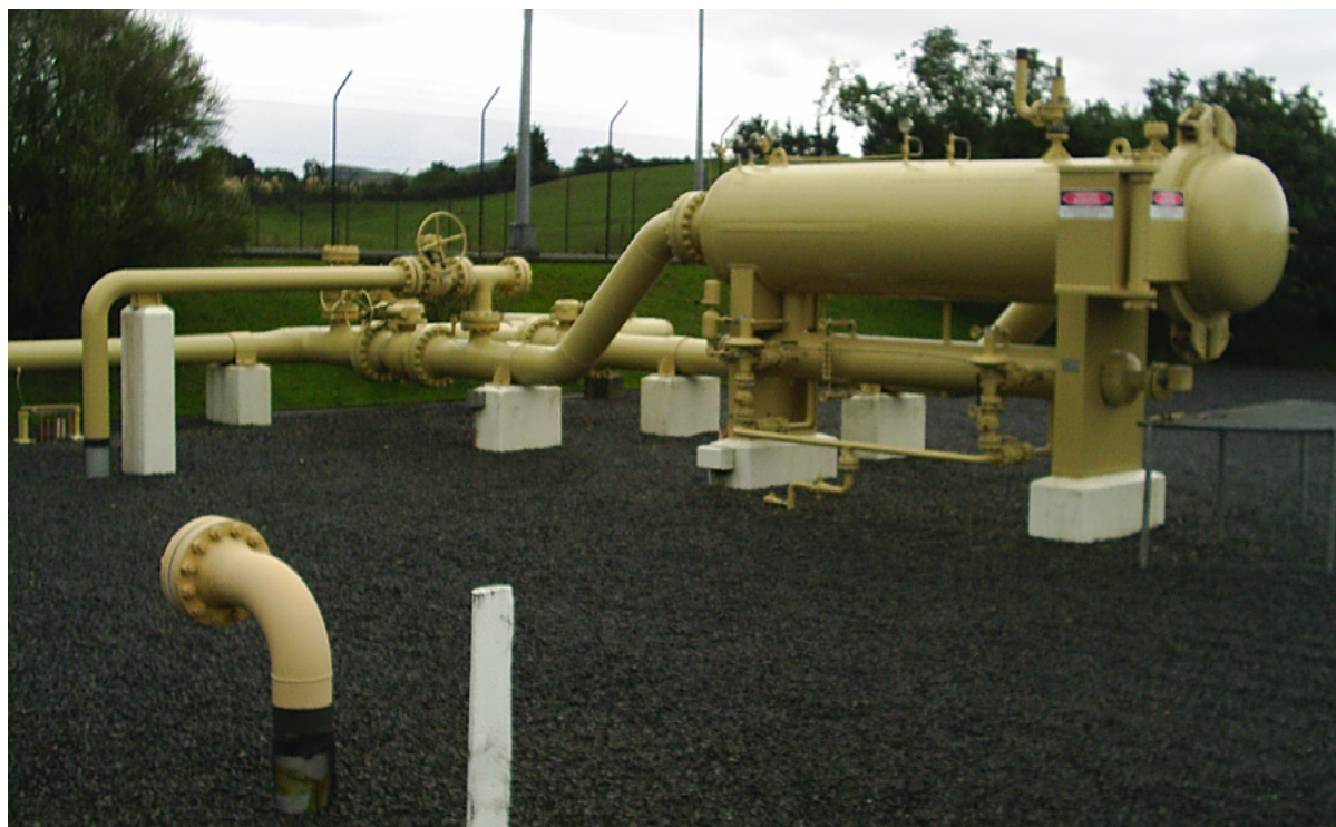
Figure 28: Typical filter separator
