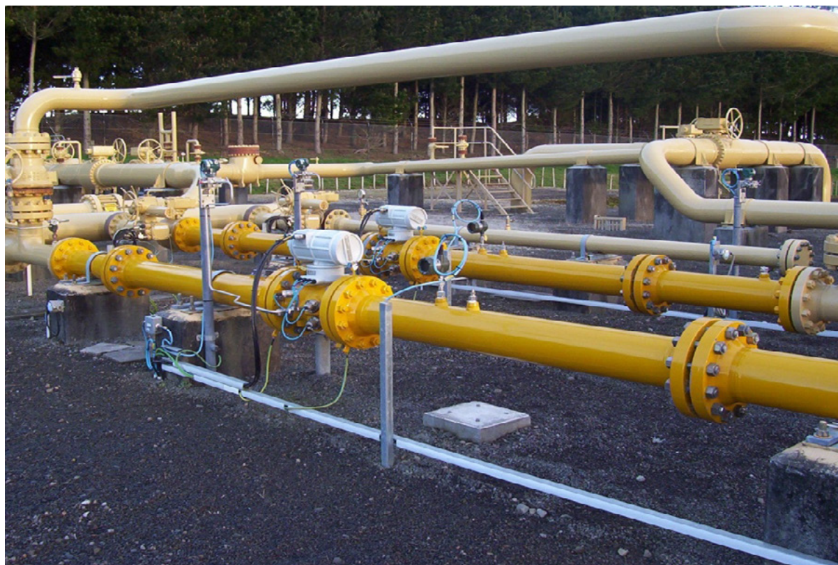
Figure 32: Typical Ultrasonic Metering System
