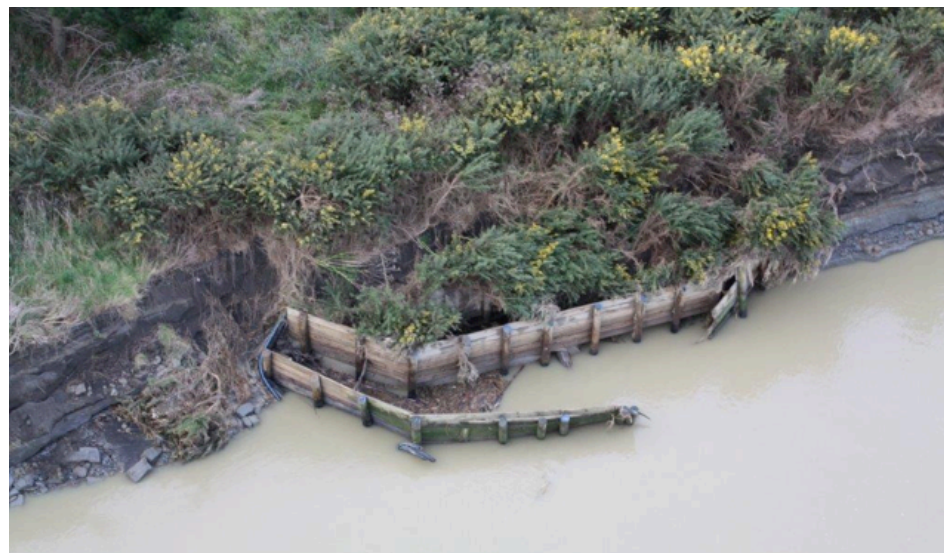
▲ The photograph above is of the existing Turakina river bank protection.
