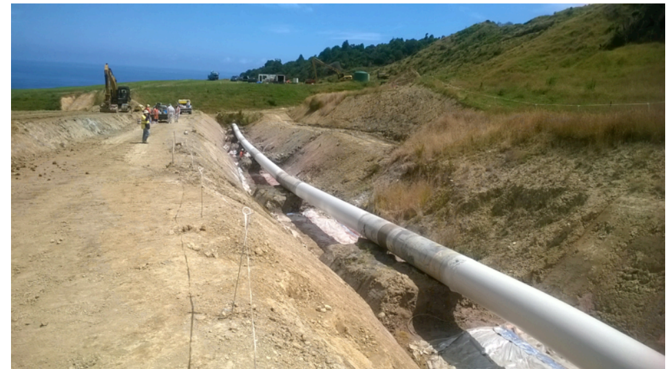
▲ The photo above is an example of recoating work being conducted on First Gas assets.
